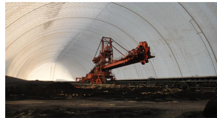
Bulk Material Storage
